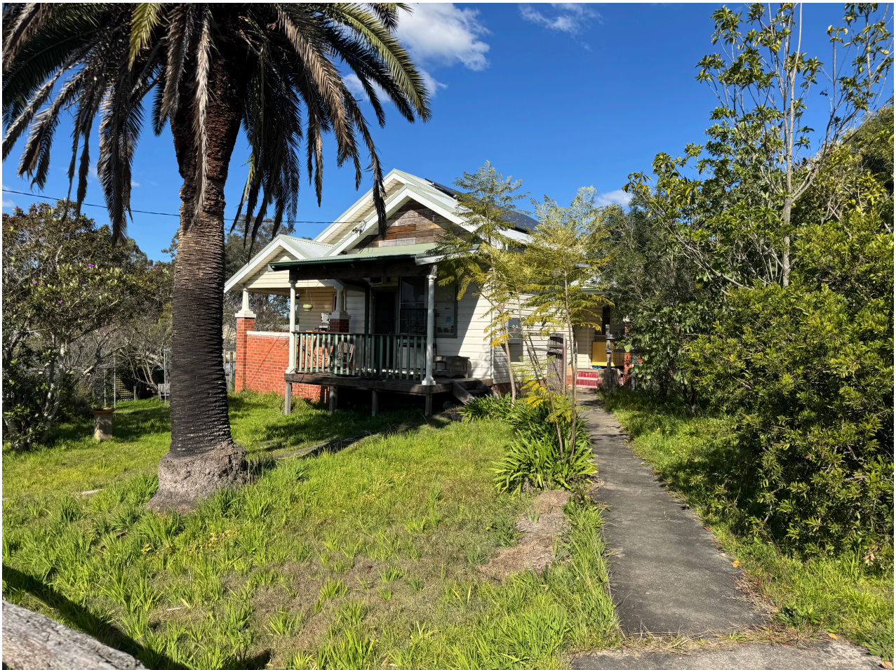
Figure 1 Site viewed Myles Street
